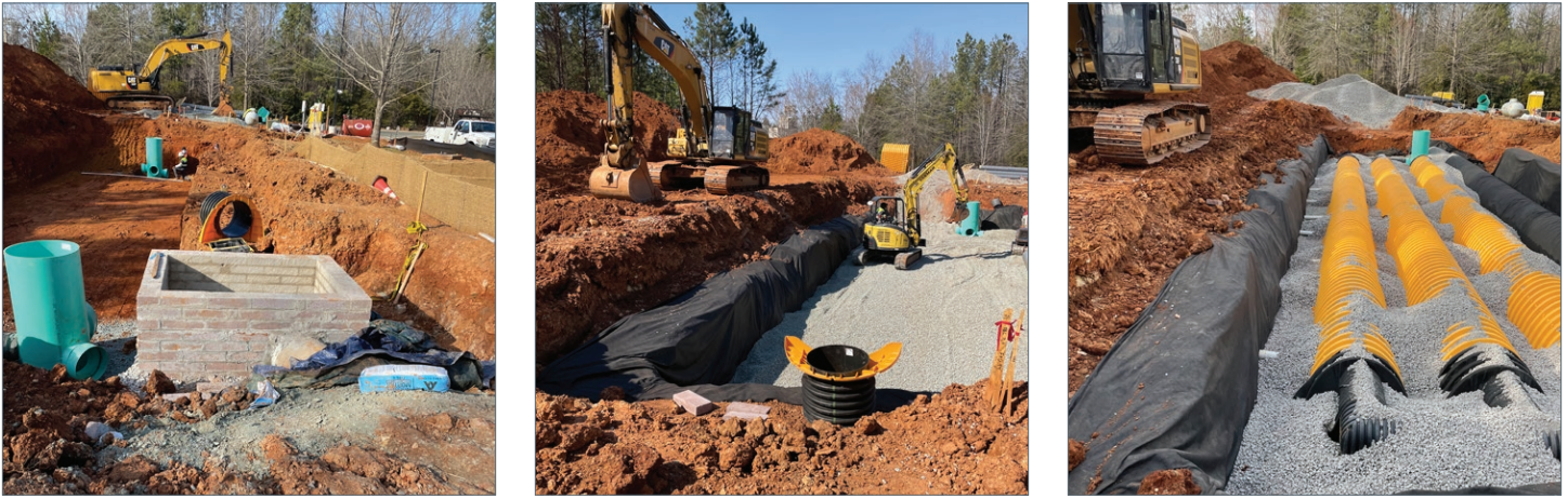
Figure 2. Construction phases of a perforated pipe type underground stormwater detention system.
