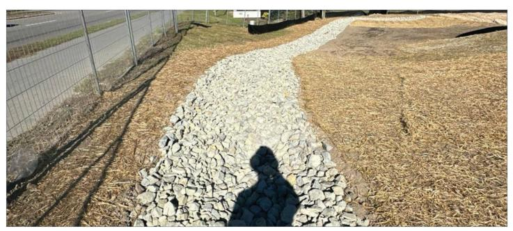
Riprap channels are a widely used erosion control solution that provides stability to embankments, channels, and shorelines. By employing stone or other durable materials, riprap serves as a natural and effective way to manage water flow and prevent erosion. This document explores the purpose, function, design, and implementation of riprap channels for both large-scale infrastructure and smaller civil engineering projects.
